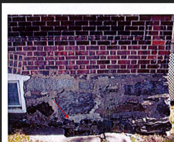
Fig. 5: Emptied mortar joints at foundation walls in expanding massive masonry.
