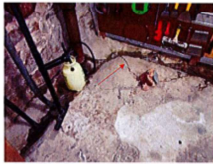
Fig. 7: The concrete binding slab in the basement of the old part of the building is cracked.
