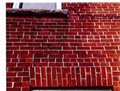
Fig. 30: Crack in the 1900's wall.
