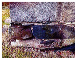
Fig. 6: Fissured and emptied mortar joints at the west corner of the foundation walls.
