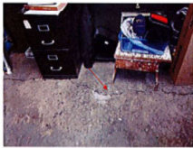
Fig. 8: More cracks in the concrete slab.
