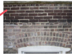
Fig. 40: Certain areas of masonry were repointed at an unknown date. The mortar used has a high Portland cement content which is not compatible with the old masonry of the building.
