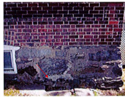
Fig. 5: Emptied mortar joints at foundation walls in expanding massive masonry.
