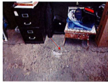
Fig. 8: More cracks in the concrete slab.
