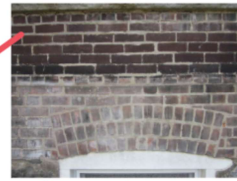
Fig. 40: Certain areas of masonry were repointed at an unknown date. The mortar used has a high Portland cement content which is not compatible with the old masonry of the building.
