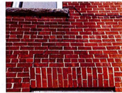
Fig. 30: Crack in the 1900's wall.
