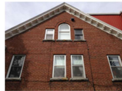
Fig. 84: Wooden gullotine windows with aluminum storm windows at the upper levels which are obviously not original.
