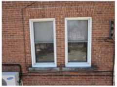
Fig. 85: Most recent windows with PVC-clad exterior on the north-east façade.
