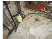
Fig. 7: The concrete binding slab in the basement of the old part of the building is cracked.
